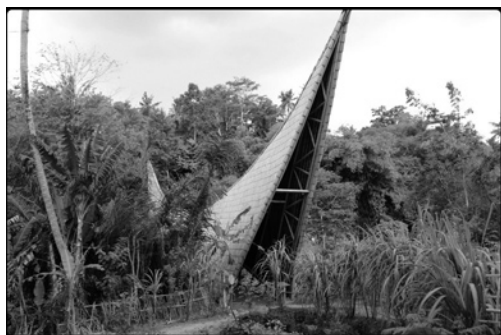
This bamboo bridge in the Green School is built without any additional material. Just bamboo.
